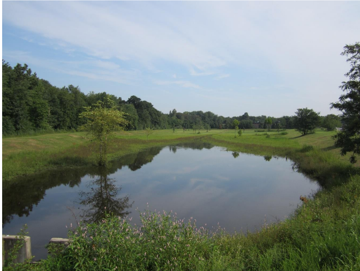
Standing water in detention basin
