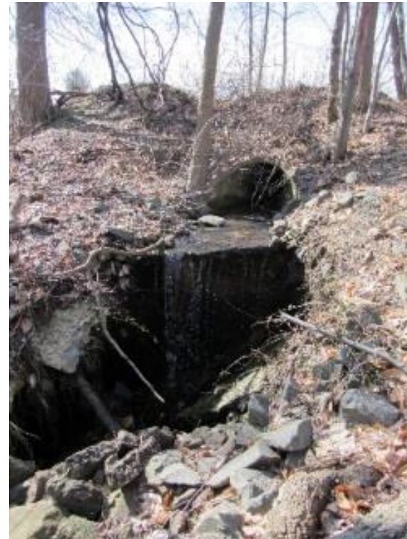
Outlet Destabilization
